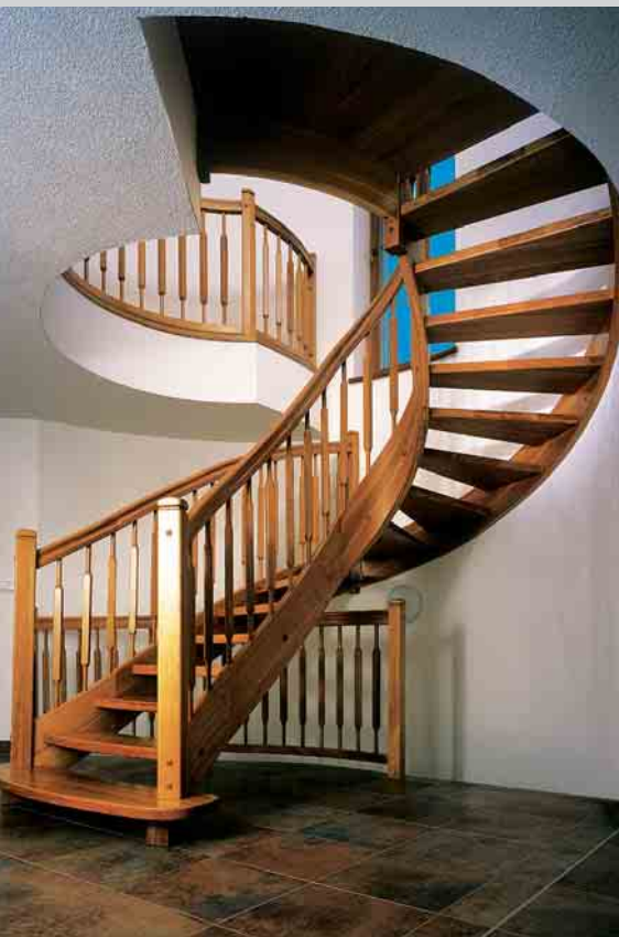
Mortised String Staircase
